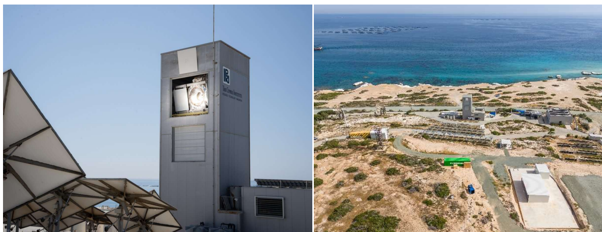
The solar receiver tower and a view across the facility and the coastline.
